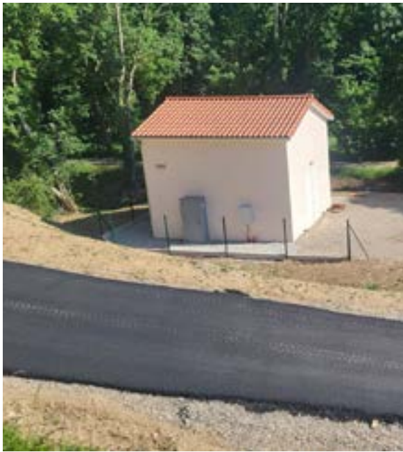
Station de pompage D1082
